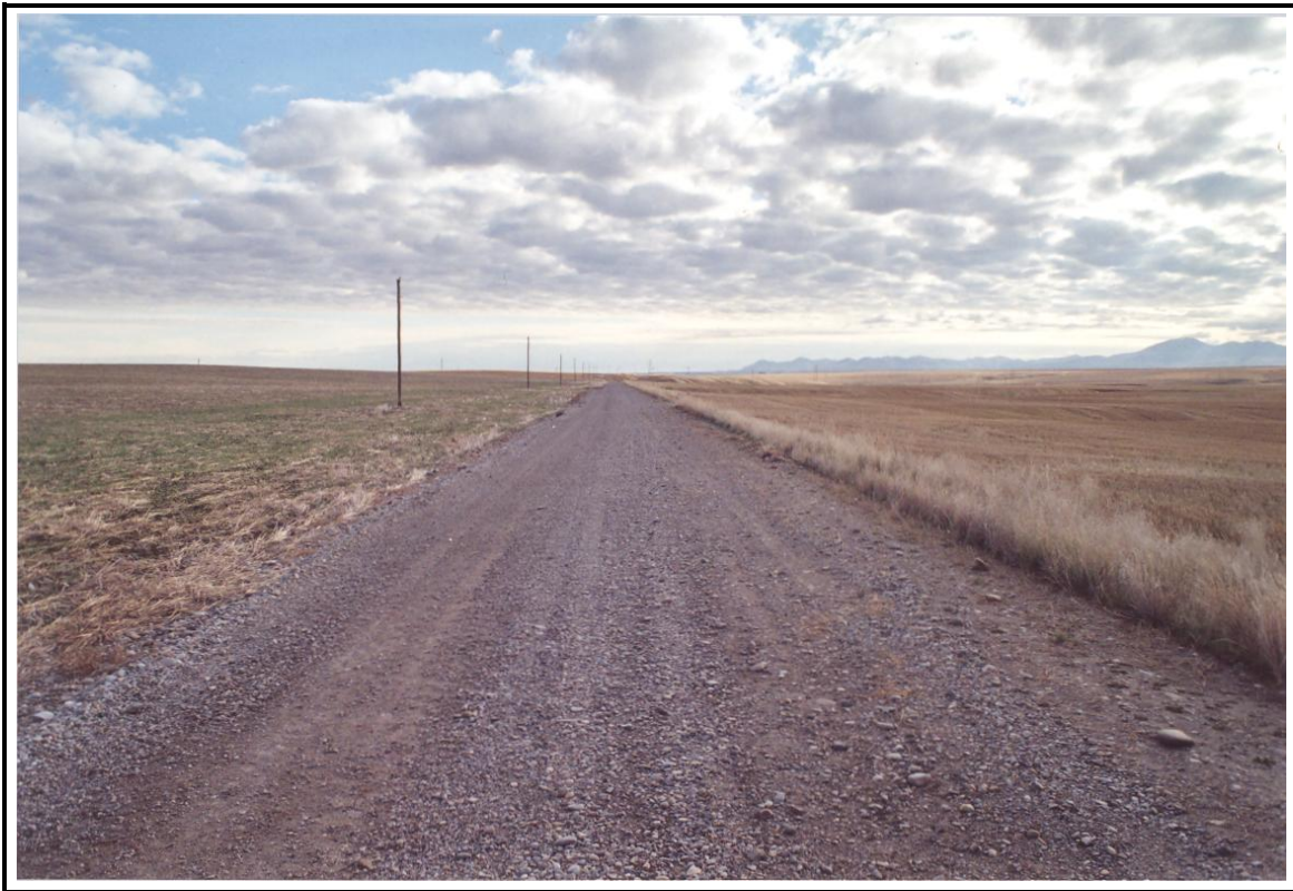
Figure 10. Typical graded and gravel-surfaced section of 24CA264. View to the east/northeast.
