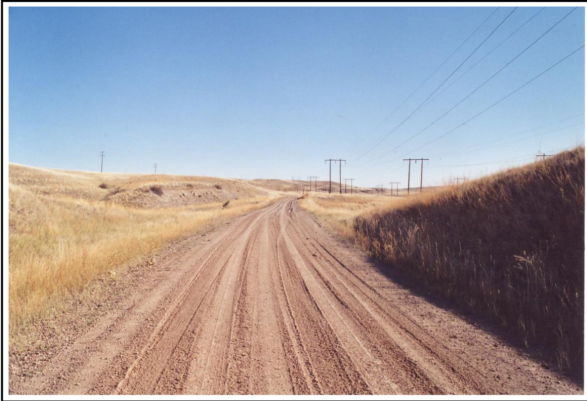
Figure 14. Section of the 24CA416 road located midway between the Rainbow and Ryan hydroelectric facilities. View to the Northeast.
