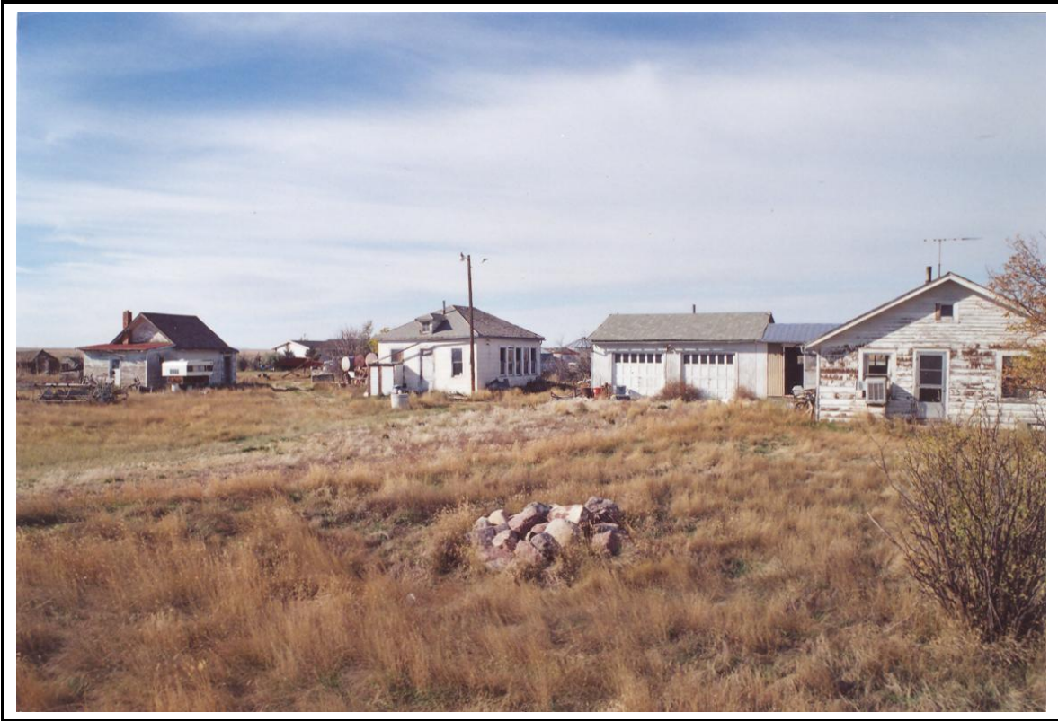
Figure 22. Overview of the Kantola Farmstead (24CA988) from Salem Road. View to the west/southwest.
