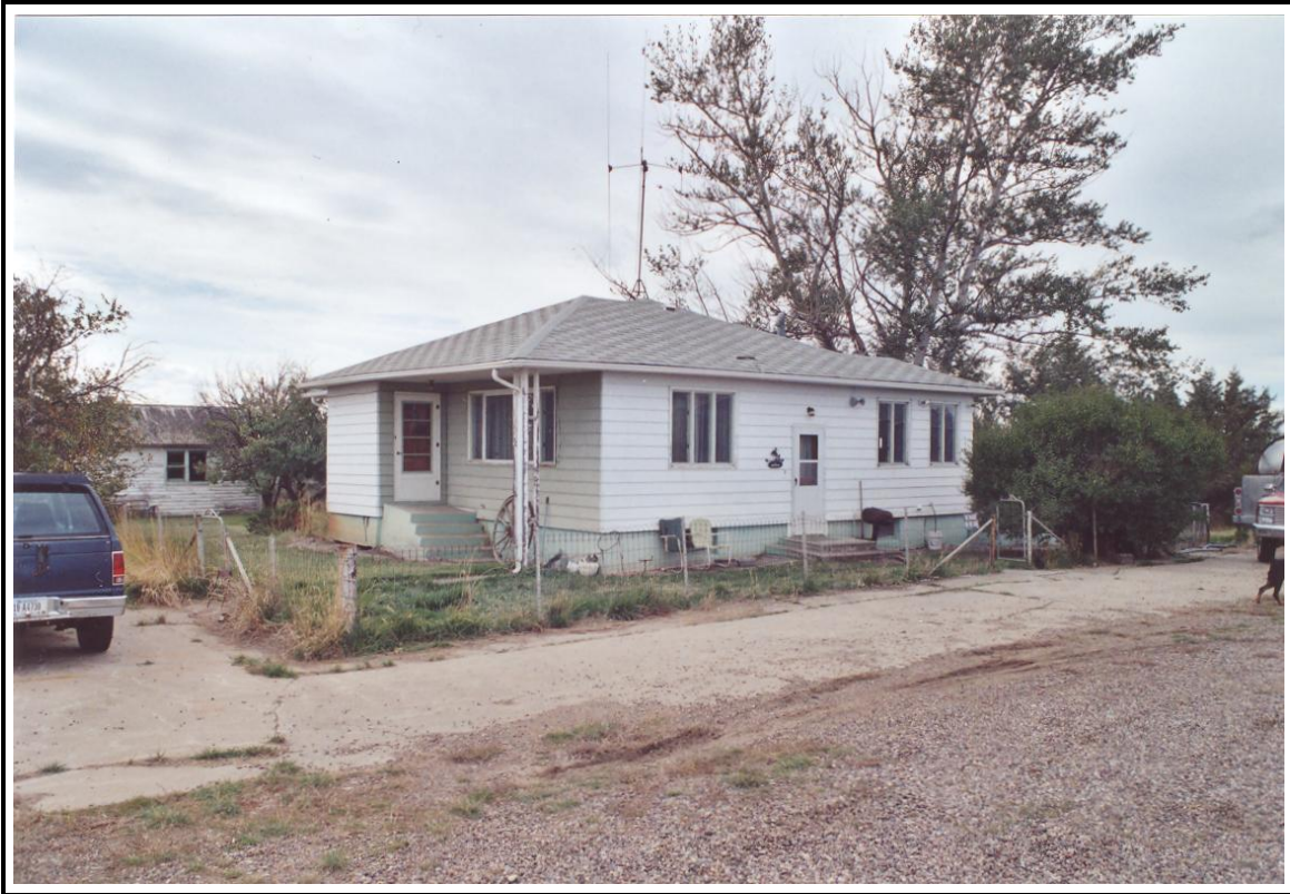
Figure 17. The Feature 1 house at 24CA986. View to the southwest.
