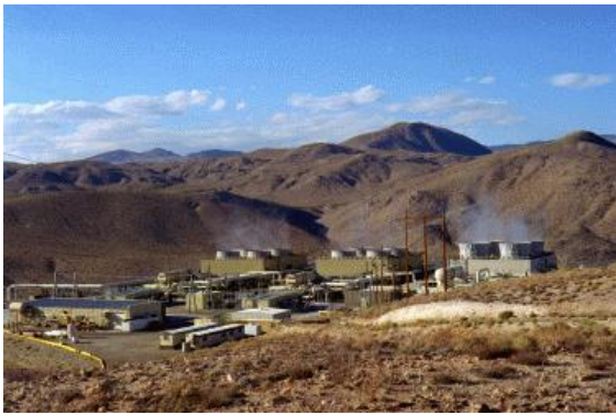
Figure 2-12. CalEnergy Navy I Flash Power Plant at the Coso Geothermal Field in California (85 MW net capacity)
