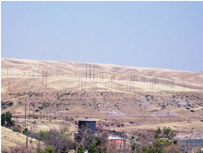
Figure 3-51. 230 kV Transmission Lines Prominent Element in Scenery North of Missouri River and East of Great Falls Switchyard
