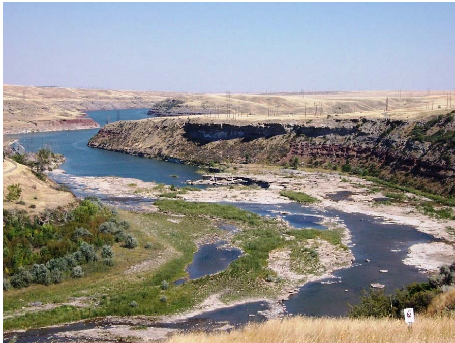
Figure 3-50. Missouri River Downstream of Rainbow Falls; Existing 230 kV Transmission Lines Visible Approaching and Spanning River
