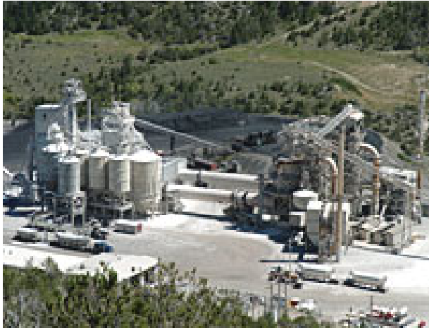
Figure 2-32. Graymont's Indian Creek Lime Plant near Townsend, MT
