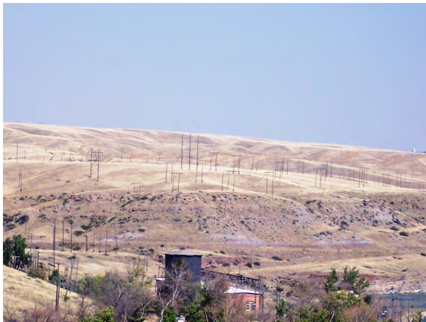
Figure 3-51. 230 kV Transmission Lines Prominent Element in Scenery North of Missouri River and East of Great Falls Switchyard
