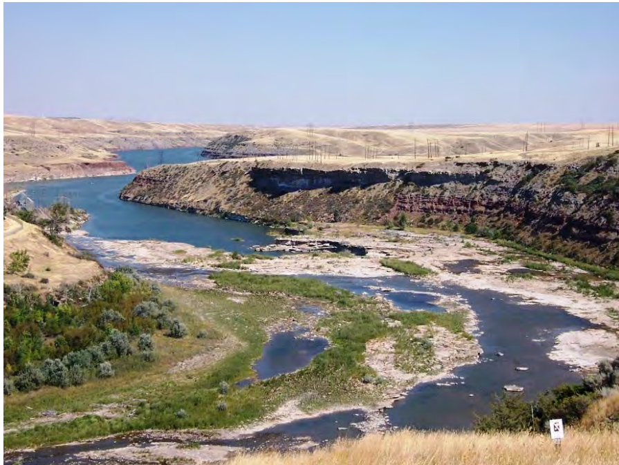
Figure 3-50. Missouri River Downstream of Rainbow Falls; Existing 230 kV Transmission Lines Visible Approaching and Spanning River
