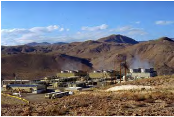
Figure 2-12. CalEnergy Navy I Flash Power Plant at the Coso Geothermal Field in California (85 MW net capacity)
